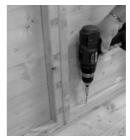
4 Fix to floor using 2 x 60mm screws per panel
