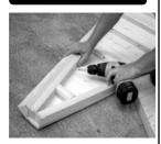
1 Secure one angled post to the same side of each panel using 3 x 60mm screws per post. Make sure the square end of the post is at the top of the panel and level with the top of the studwork.
