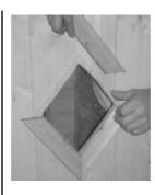
3 Slide in the glaze then fit the remaining two pieces of angled rebated strip to the top using 2 x 20 mm screws per piece. Repeat for other window.
