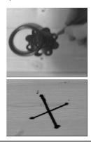
2 Fix black ring handle using 4 x 25mm black screws. Place the D shaped handle on the inside of the door and fix using 4 x 25 mm black screws.
